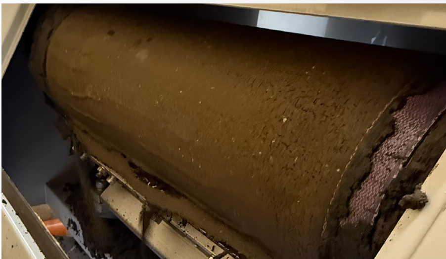
Outlet from MP-EDW
